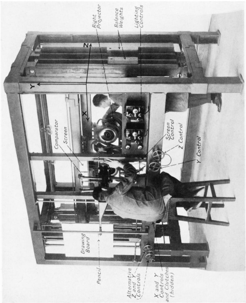
5. The Barr and Stroud Photogrammetric Plotter
